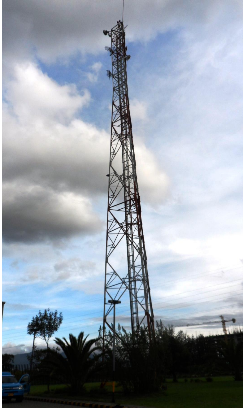
C. CONTROL MODELIA - TORRE AUTOSOPORTADA 40 M - TRIANGULAR
