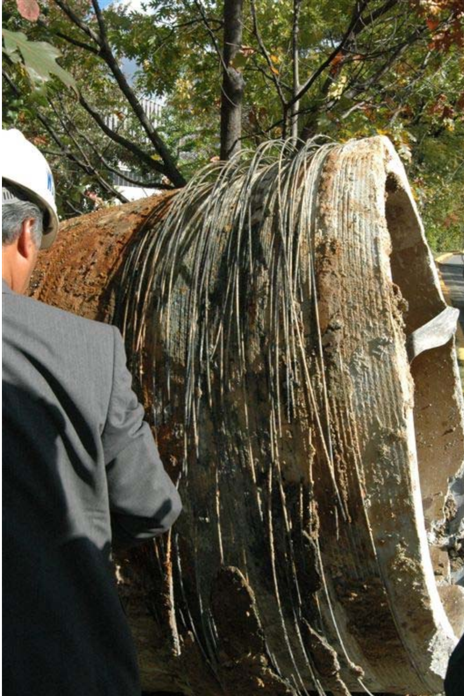
Wire Break Damage on the bell portion of the pipe section.
