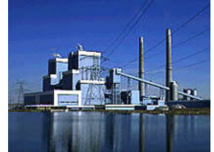
Figure 1 Antelope Valley Station
