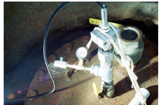
Figure 2 PPIC's hydrophones can be installed through valves as small as 1" in diameter
